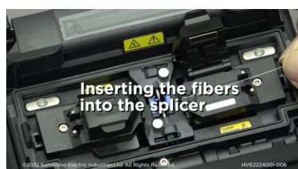
Inserting the fibers into the splicer
